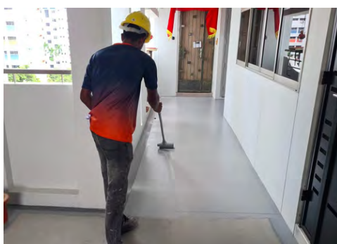
PU Coating Application @ Common Areas
